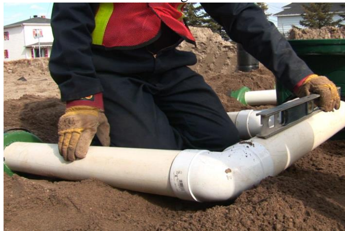
Fig. 76 – Feed Pipe sloped toward Advanced Enviro-Septic ®
