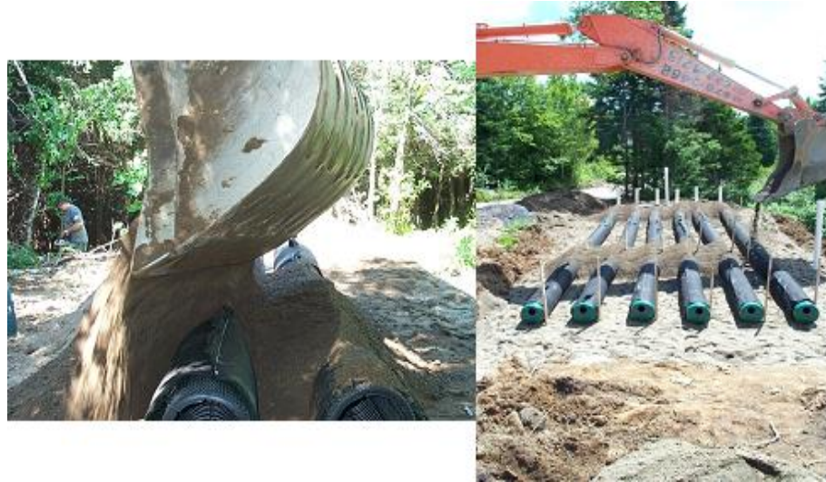
Fig. 65 – Covering the Advanced Enviro-Septic® pipes
