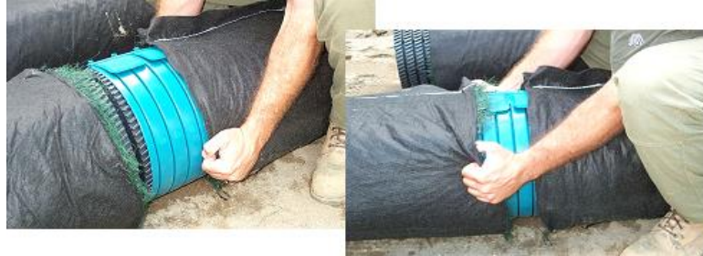
Fig. 61 – Replacing the membranes over the coupling
