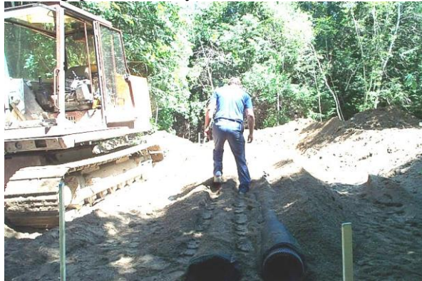
Fig. 66– Filling the void around the Advanced Enviro-Septic® pipes
