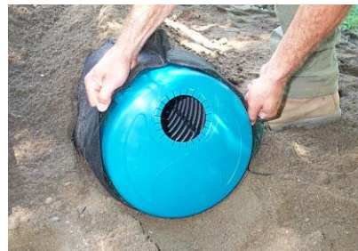
Fig. 62 – Installation of the single offset adapter
