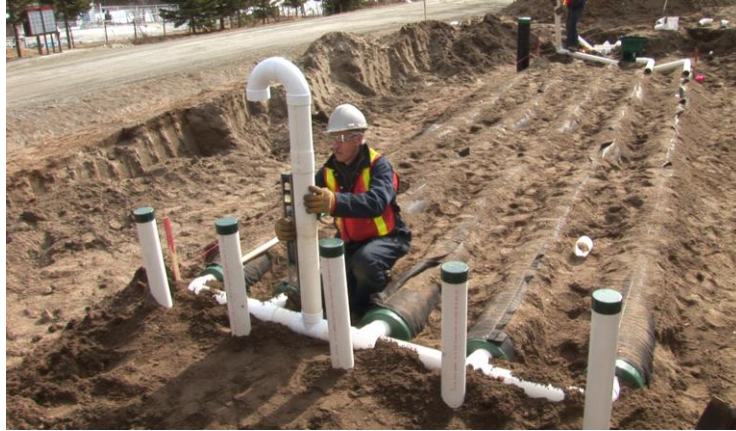
Fig. 69 – Aeration pipe and vent installation
