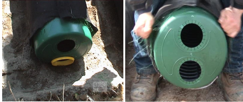
Fig. 63 - Installation of the double offset adapter (old and new style)
