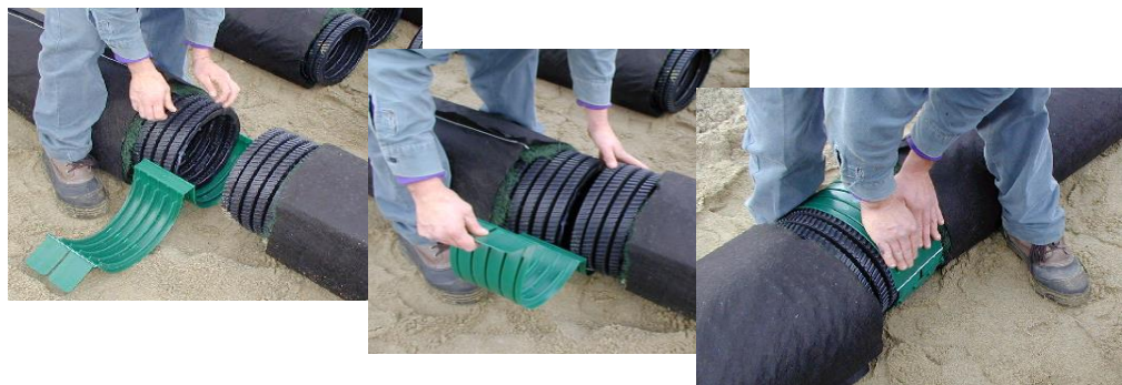
Fig. 60 – Coupling installation
