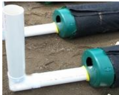
Fig. 68 – Piezometer installation
